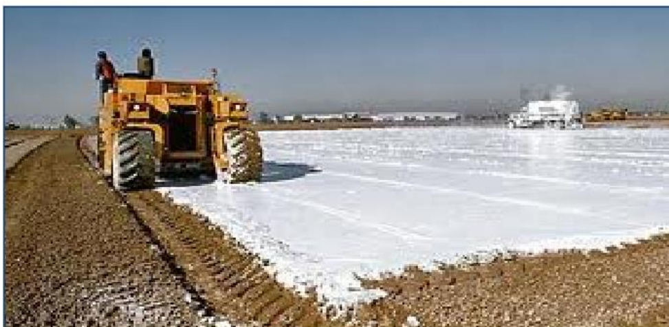
Figure 1. Application of Lime Stabilization (Mukherjee, 2014)
